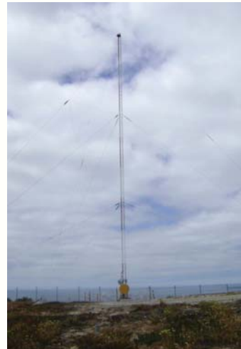
NDB da Caparica LAT:38°38'32"N LONG:09°13'17"W Emissor– 389 KHz, 1 KW
